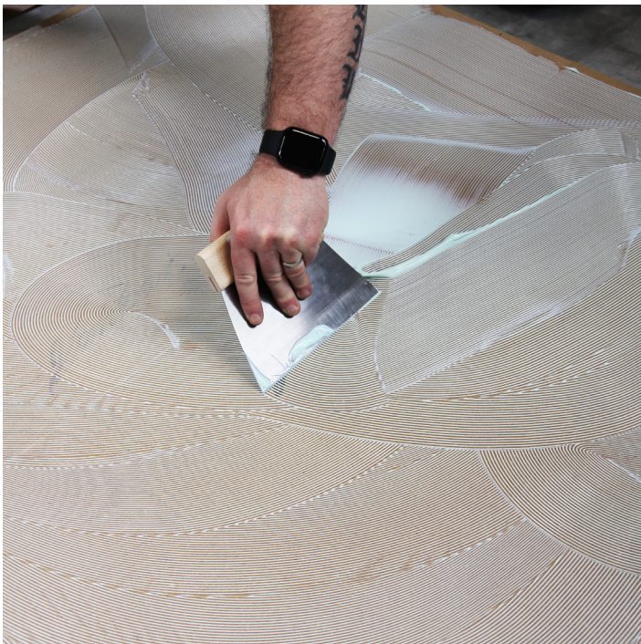
Applying the adhesive to the subfloor
