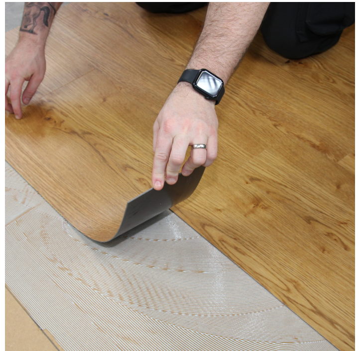
Applying the flooring into the adhesive
