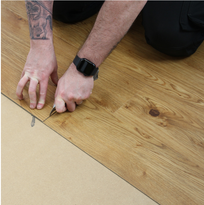
Marking and scoring for cuts
