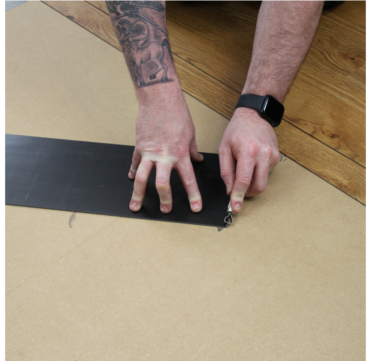
Removing the BUR and applying the micro bevel
