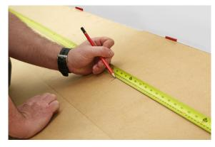
Measure from wall to wall and ensure that you start installing in a logical place to minimise any cut planks to the perimeter of the installation. Mark a "starting line" on the floor with your pencil. Ensure that you include the 5mm expansion gap when measuring. More information in the detailed fitting instructions in each box.
