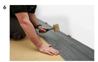
Once you have positioned each "short end" into place, gently tap the top surface of the plank using a rubber mallet (from a height of approx 10cm above the surface) to engage locking system. The surfaces of the planks should be perfectly flush after tapping down. Do not use extra force and never use a solid tool such as a metal hammer as this could cause damage to the joint.
