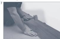
Once you have positioned each "short end" into place, gently tap the top surface of the plank using a rubber mallet (from a height of approx 10cm above the surface) to engage locking system. The surfaces of the planks should be perfectly flush after tapping down. Do not use extra force and never use a solid tool such as a metal hammer as this could cause damage to the joint.
