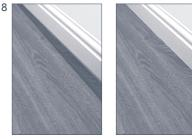
Now your floor is fully installed, you can replace your skirting boards. Be careful not to fully trap the flooring as it needs to be able to expand and contract freely. Usually 1-2mm is enough to allow this to happen. If you left the skirting boards on, then use Scotia beading to cover your Smm expansion gap. Never use any type of filler to cover your expansion gap.
