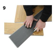
To engage the system correctly click sides are locked into place. You Preparation' may wish to use a rubber mallet and tapping block to assist with this.
