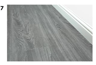
Now your floor is fully installed, you can replace your skirting boards. Be careful not to fully trap the flooring as it needs to be able to expand and contract freely. Usually 1-2mm is enough to allow this to happen. If you left the skirting boards on, then use Scotia beading to cover your 5mm expansion gap. Never use any type of filler to cover your expansion gap.
