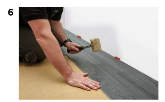
Once you have positioned each "short end" into place use a rubber mallet to tap the drop lock system into action. This should be done on every short end joint. The long ends do not require any additional force to lock into position.
