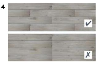
When planning where to start from, ensure that you stagger the joints on each row. There should be at least a 1/3rd of a plank or tile length between each end joint. Do not have all the joints running in a line.
