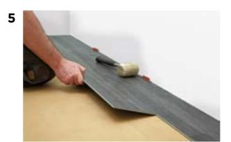
Start the installation by angling each plank into the click locking system along the long ends and then lay each plank flat to the floor. The long ends have a click lock system to hold each plank in place. The short ends have a drop lock system..
