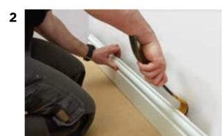
A 5mm expansion gap is needed around the entire perimeter of the flooring. You may wish to remove the skirting boards and replace after installation or use Scotia beading to cover the expansion gap. In this instance we have removed the skirting boards.
