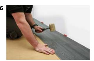
Once you have positioned each "short end" into place use a rubber mallet to tap the drop lock system into action. This should be done on every short end joint. The long ends do not require any additional force to lock into position.
