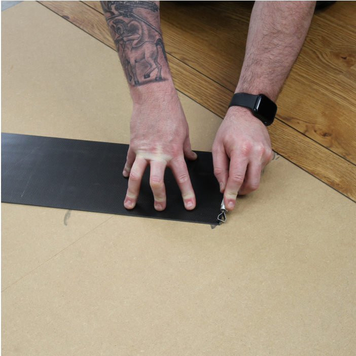
Removing the BUR and applying the micro bevel
