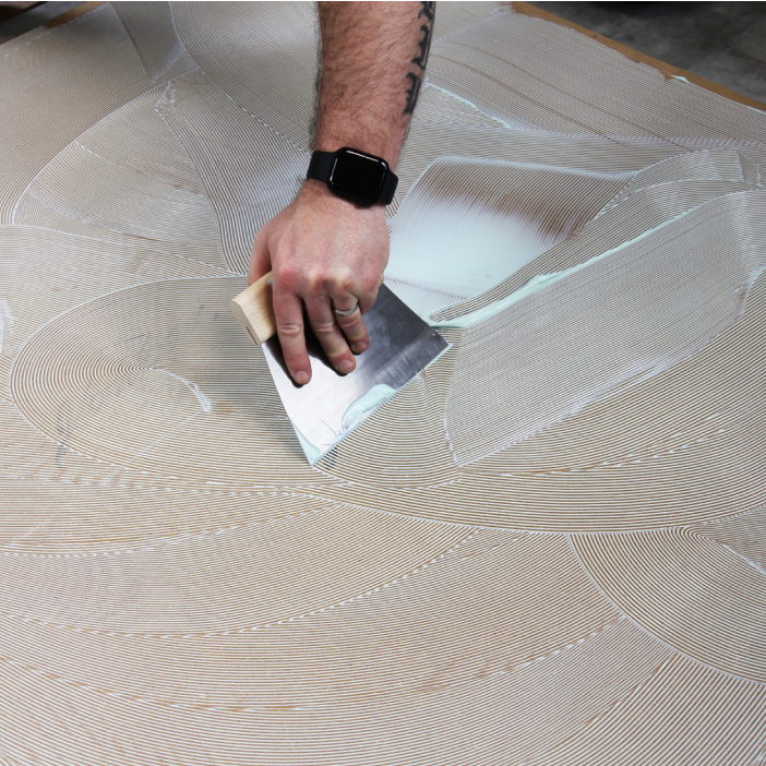
Applying the adhesive to the subfloor
