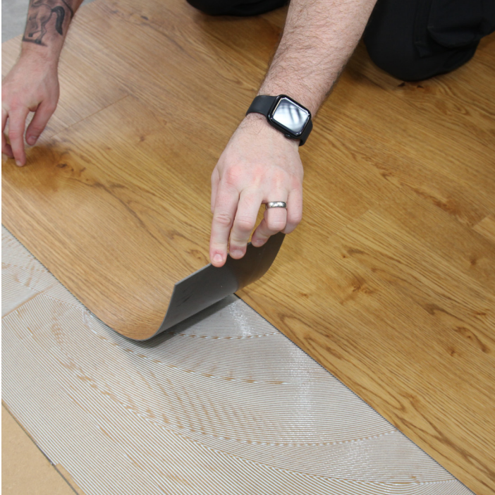
Applying the flooring into the adhesive
