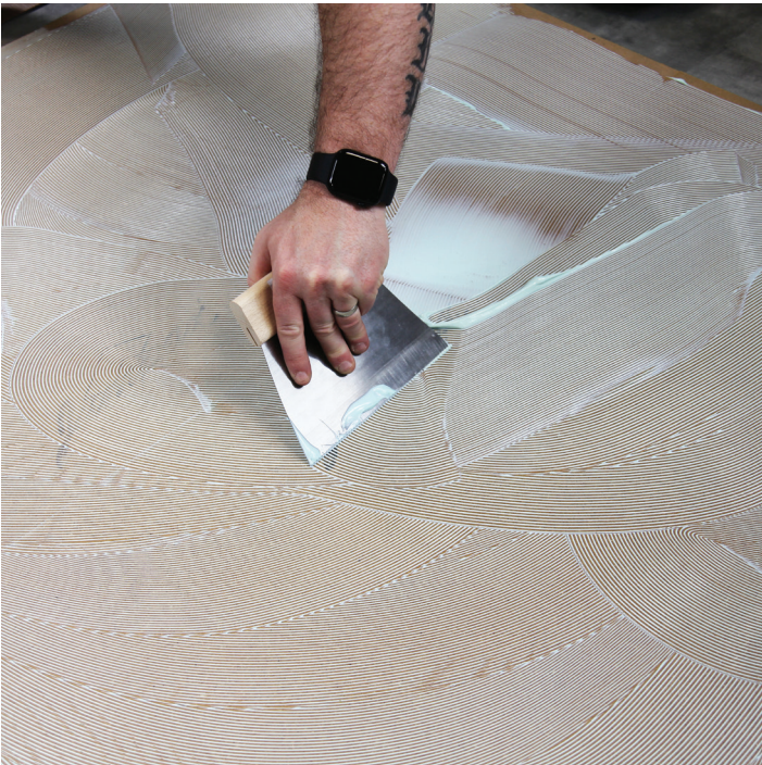
Applying the adhesive to the subfloor
