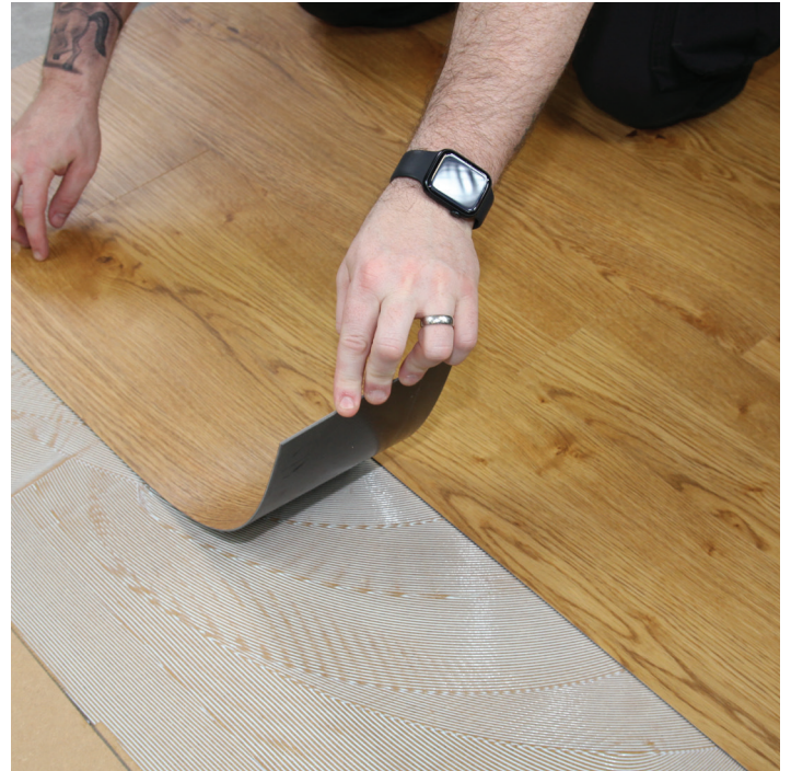
Applying the flooring into the adhesive
