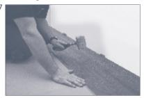
Once you have positioned each "short end" into place, gently tap the top surface of the plank using a rubber mallet (from a height of approx 10cm above the surface) to engage locking system. The surfaces of the planks should be perfectly flush after tapping down. Do not use extra force and never use a solid tool such as a metal hammer as this could cause damage to the ioint.
