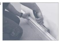
A 5mm expansion gap is needed around the entire perimeter of the flooring. You may wish to remove the skirting boards and replace after installation or use Scotia beading to cover the expansion gap. In this instance we have removed the skirting boards.
