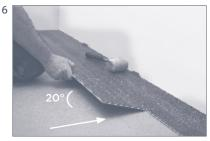
Start the installation by angling each plank into the click locking system along the long ends and then lay each plank flat to the floor. The long ends have a click lock system to hold each plank in place. The short ends have a drop lock system. More details in the detailed fitting instructions.
