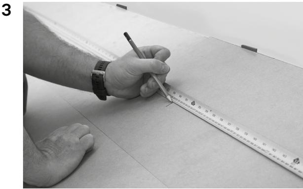
3 Measure from wall to wall and ensure that you start installing in a logical place to minimise any cut planks to the perimeter of the installation. Mark a “starting line” on the floor with your pencil. Ensure that you include the 5mm expansion gap when measuring.
