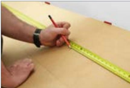
Measure from wall to wall and ensure that you start installing in a logical place to minimise any cut planks to the perimeter of the installation. Mark a "starting line" on the floor with your pencil. Ensure that you include the 5mm expansion gap when measuring. More information in the detailed fitting instructions in each box.
