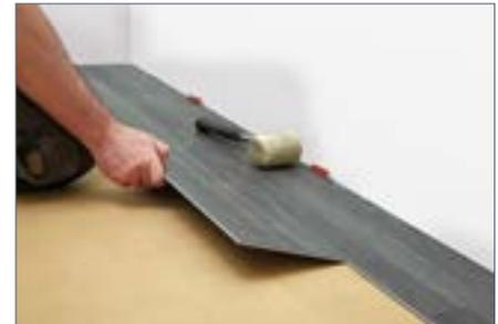
Start the installation by angling each plank into the click locking system along the long ends and then lay each plank flat to the floor. The long ends have a click lock system to hold each plank in place. The short ends have a drop lock system. More details in the detailed fitting instructions.
