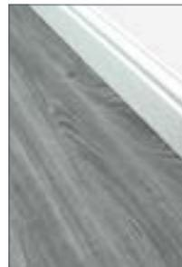
Now your floor is fully installed, you can replace your skirting boards. Be careful not to fully trap the flooring as it needs to be able to expand and contract freely. Usually 1-2mm is enough to allow this to happen. If you left the skirting boards on, then use Scotia beading to cover your 5mm expansion gap. Never use any type of filler to cover your expansion gap.
