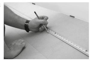
Measure from wall to wall and ensure that you start installing in a logical place to minimise any cut planks to the perimeter of the installation. Mark a "starting line" on the floor with your pencil. Ensure that you include the 5mm expansion gap when measuring.
