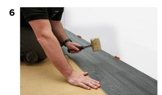
To start the 2nd row, position the drop lock joint of the panel over the joint of the panel in the 1st row and tap into place using a rubber mallet. Again, take care to ensure the joints are perfectly aligned before tapping into place. Continue the 2nd row by angling the tongue of the 2nd panel into the groove of the 1st panel and tapping the drop lock joint into the adjacent panel of the 1st row. Repeat the process until all rows are installed.
