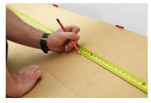
Measure from wall to wall and ensure that you start installing in a logical place to minimise any cuts across the panels to the perimeter of the installation. Mark a "starting line" on the floor with your pencil. Ensure that you include the 5mm expansion gap when measuring.
