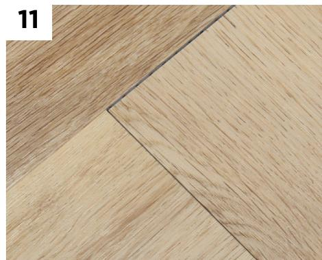
Should your floor look like the example above, the system has not engaged correctly due to either the plank not being locked together perfectly or the subfloor being out of tolerance, not necessarily at the point detected in the visible joint. You may need to backtrack over the install to detect the error.
