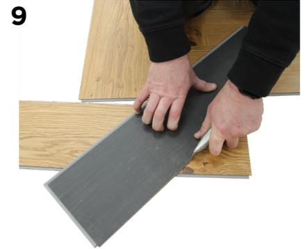
To cut the product use sharp knife like the one shown in this diagram. You can use a plank as a ruler / guide to cut along. Keep your off cuts as they may become useful for finishing around the perimeter.
