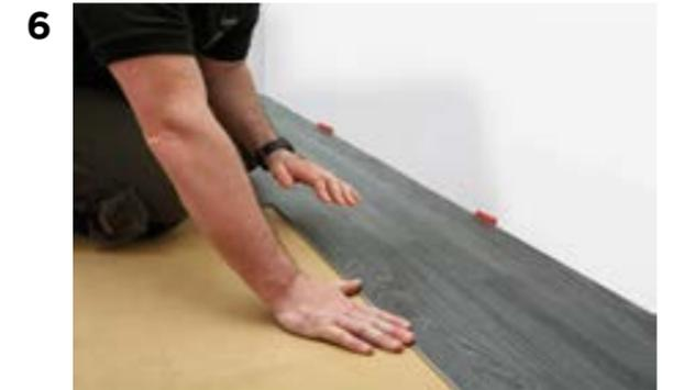
Click the "short end" joints together by angling the tongue into the groove of the next piece and dropping it flat to lock the joint. The short end joint should be locked together first and then the long end joint into the previous row.
