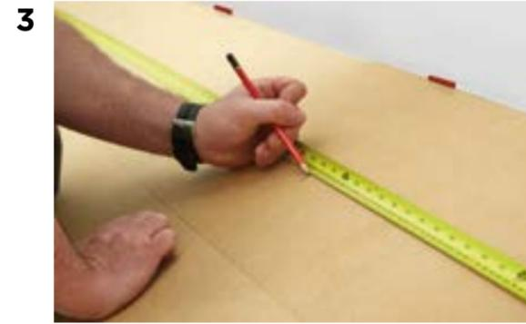
Measure from wall to wall and ensure that you start installing in a logical place to minimise any cut planks to the perimeter of the installation. Mark a "starting line" on the floor with your pencil. Ensure that you include the 5mm expansion gap when measuring.
