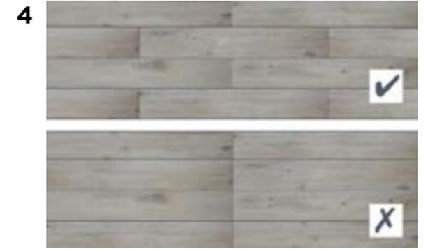
When planning where to start from, ensure that you stagger the joints on each row. There should be at least a 1/3rd of a plank or tile length between each end joint. Do not have all the joints running in a line.
