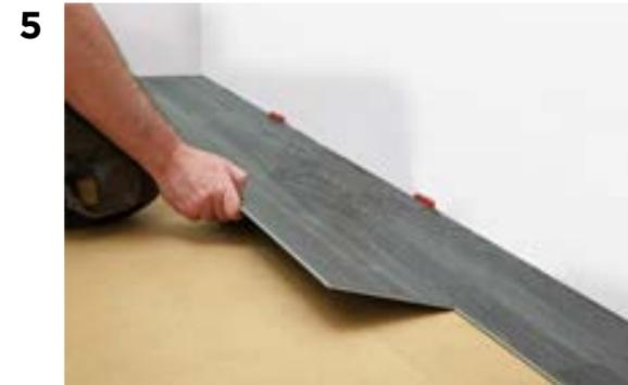
Start the installation by angling each plank into the click locking system along the long ends and then lay each plank flat to the floor. The long and short ends have a click lock system to hold each plank in place.
